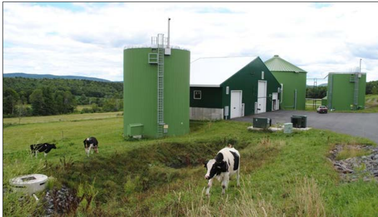
"Big Bertha" is an anaerobic digester that uses a combination of manure and organic matter to generate electricity. Image source: Vermont Technical College.
