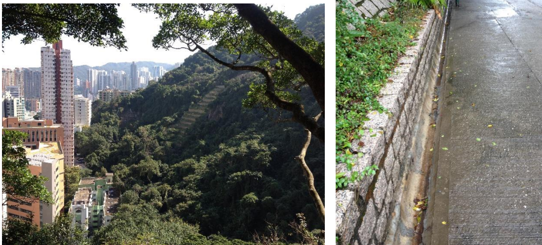
Photo of Landslide Prevention Terracing and Drainage Gutters along Hong Kong's Slope Photo by Joanna Lewis, Hong Kong, December 2013.
